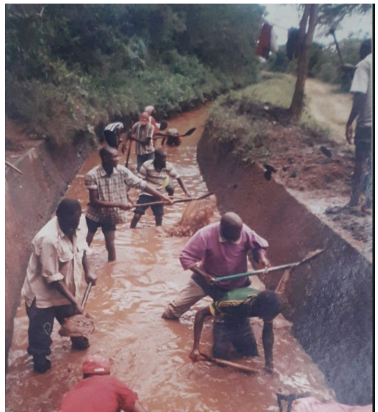
▲ Leading fellow users to manually desilt the vital Yatta Canal which is the lifeline of a large part of Yatta (2013)
